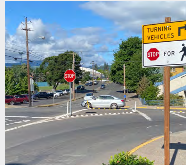
The topography at May St and 13th St creates visibility challenges. Cars traveling south through the intersection may not see pedestrians until they reach the crest of the hill, just before the crosswalk.
