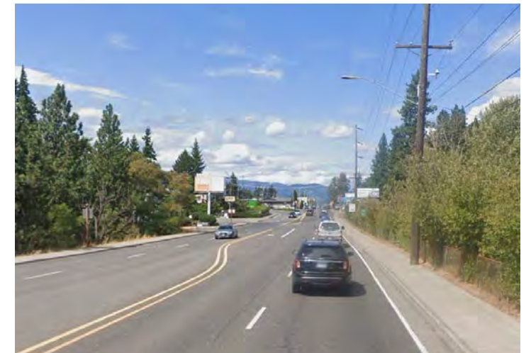
Existing Conditions at 12th St looking North toward Nix Ave
