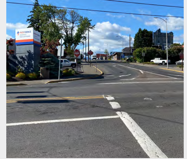
The right turn lane from 12th St onto May St has a wide curb radius, which encourages cars to enter the staggered intersection quickly. Visibility is somewhat impeded by the signs and vegetation on the southeast corner.
