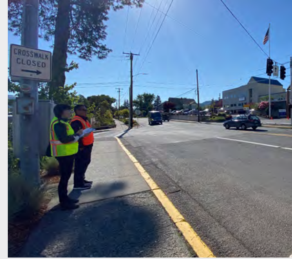
This configuration results in potential dangers for pedestrians attempting to cross 12th St at the north leg, as drivers expect to make a left turn without obstacles.
