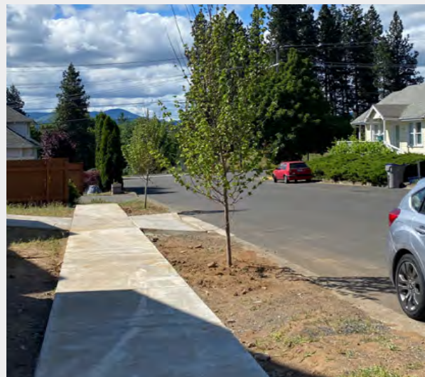
Many residential streets south of May Street Elementary have inconsistent and incomplete sidewalks.
