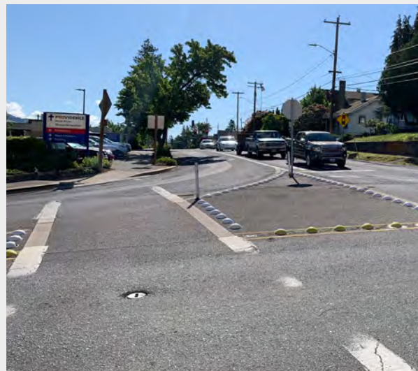
Pedestrians traveling west on May St cross a wide free right turn lane at May St and 13th St, which is built to accommodate frequent freight traffic.
