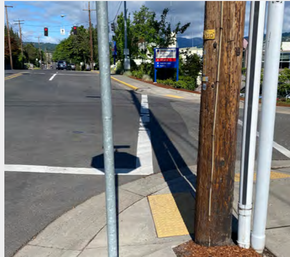
At the corner of May St and 12th St, utility poles block westbound drivers' view of pedestrians waiting to cross. At this location, the street turns from one westbound lane into two in preparation for turns.
